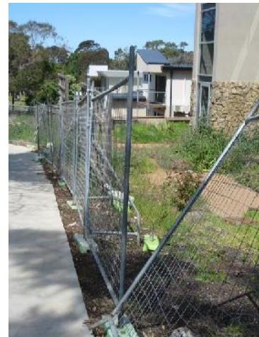
Photos show examples of unstable panels due to missing clamps and a damaged imported clamp recovered from a temporary fence in North Queensland.
