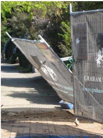
Photos show examples of unstable panels due to missing clamps and a damaged imported clamp recovered from a temporary fence in North Queensland.
